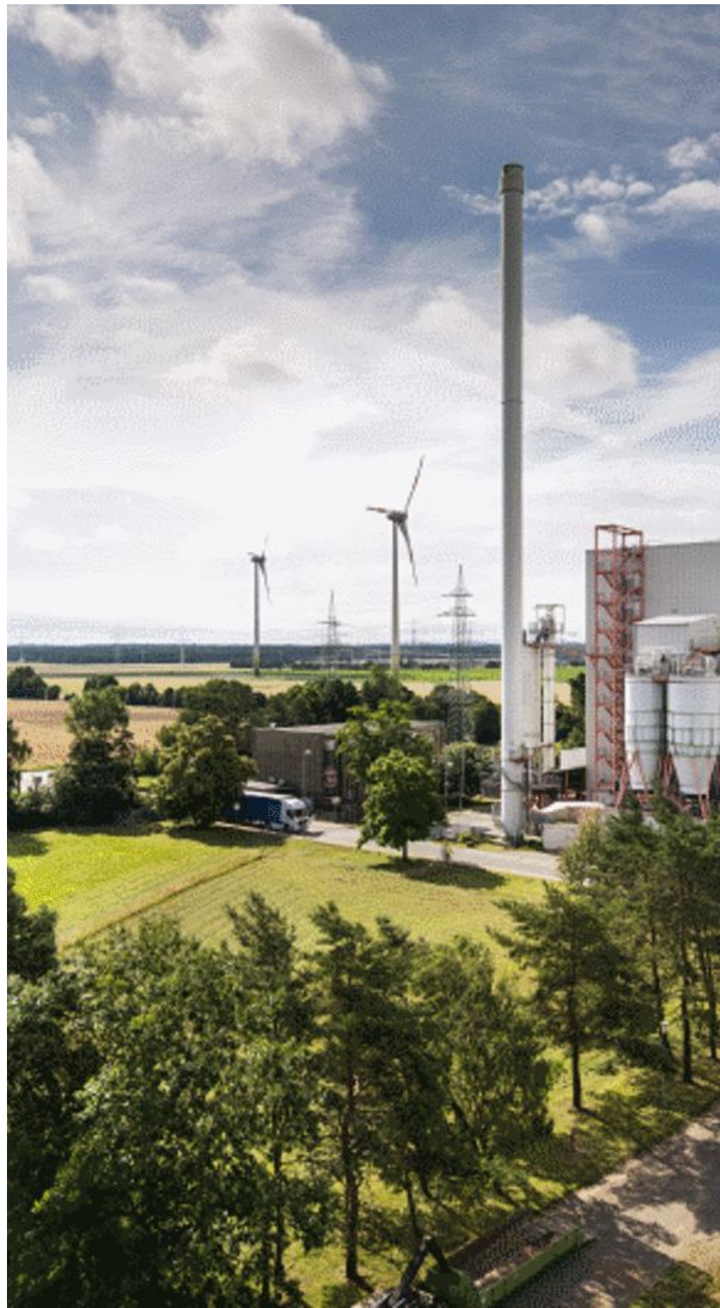
Starkraft Biomass Plant, Norway.
